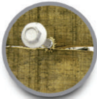
No more splitting of timber substrates
